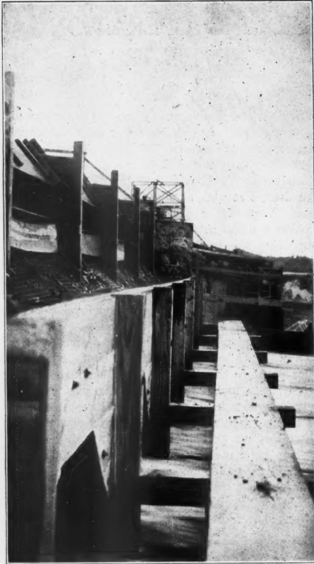
Close-up of One of the Cascades, Showing the Woven Wire Screens
